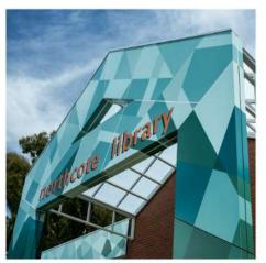
An existing library constructed in the 1980s is being refurbished to inlcude the replacement of the cladding with a decorative aluminium panel system, patterned utilising the geometry of the existing gable design.
