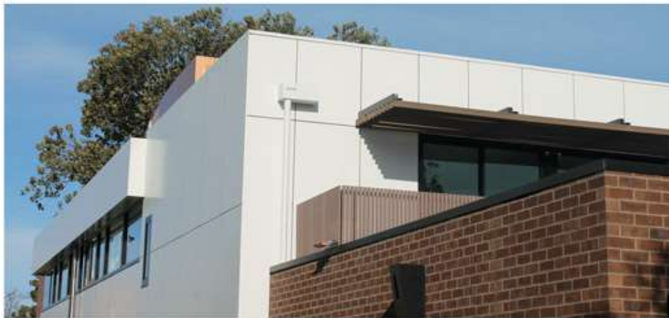
CAULFIELD NORTH APARTMENTS
